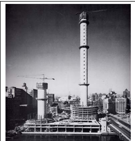
Figure 3. Marina City during construction. 1961
